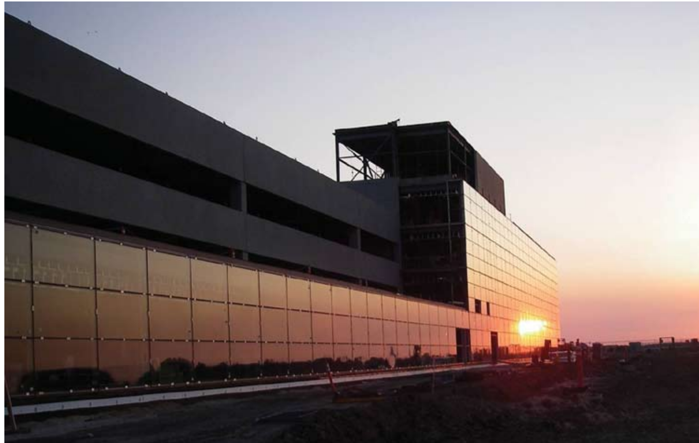
New parkade under construction, summer 2006.
