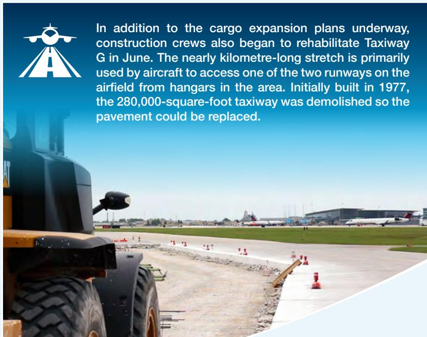
In addition to the cargo expansion plans underway, construction crews also began to rehabilitate Taxiway G in June. The nearly kilometre-long stretch is primarily used by aircraft to access one of the two runways on the airfield from hangars in the area. Initially built in 1977, the 280,000-square-foot taxiway was demolished so the pavement could be replaced.
